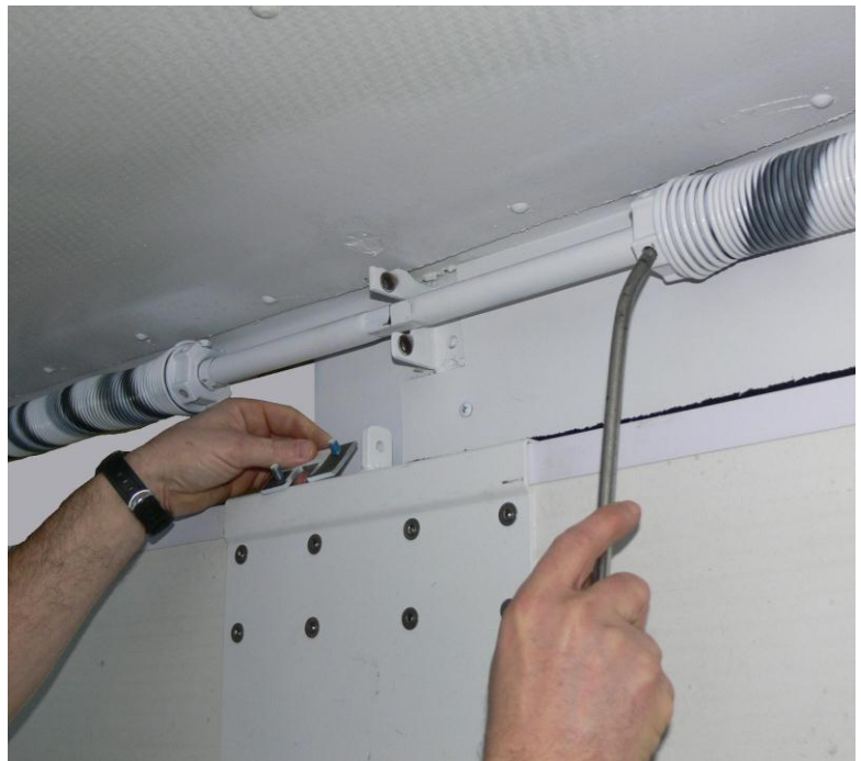
Figure 1 – Adjusting the door balancer
